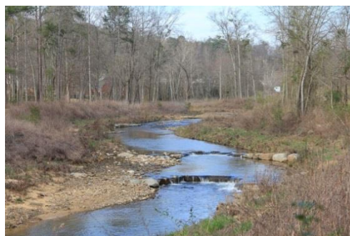
Little Shades Creek Stream Restoration Vestavia Hills
